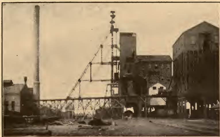
ZEIGLER MINE, ZEIGLER, ILL. OPERATED BY BELL & ZOLLER MINING CO., CHICAGO
